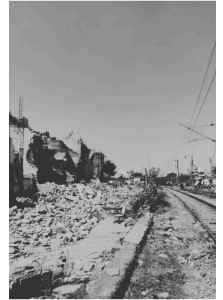
Demolition at KG Halli
